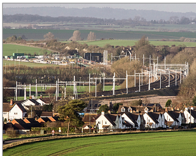
Photo caption: Electrification in progress through South Stoke
